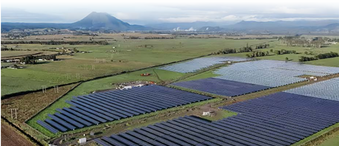
Rangitaiki - Edgecumbe Solar Farm
